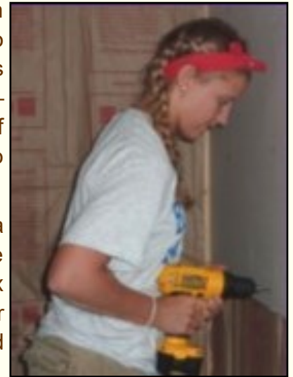
Tracy installing drywall in Dakota's soon-to-be bedroom
